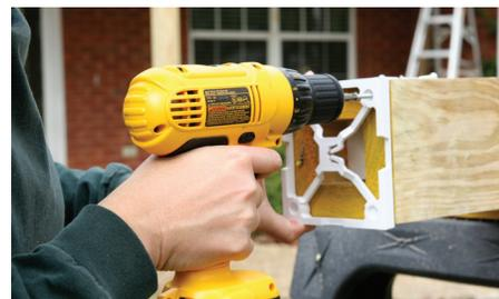
**5.** Attach plinth to the end painted yellow. This will be the bottom of your column. The factory-applied end sealant will help reduce moisture absorption.
