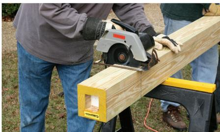
**4.** Cut using a circular saw or compound saw. Always wear protective eye wear and cut on a stable surface.
