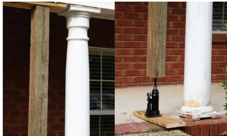
**1.** Place a temporary support next to the column you're replacing. This is accomplished with a bottle jack, a 4x4 and a 2x6. This will brace the roof line for removal of the old column and support the structure. Always be sure that the 4x4, 2x6 and related items have sufficient structural integrity to support the load.
