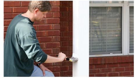
10. Prime with an oil-based primer and paint immediately. You can also stain YellaWood® columns with an oil-based stain with water-repellent.
