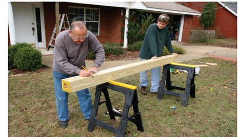
**3.** Measure new column (be sure to account for the added height of the plinth) and cut to the same length as the old.
